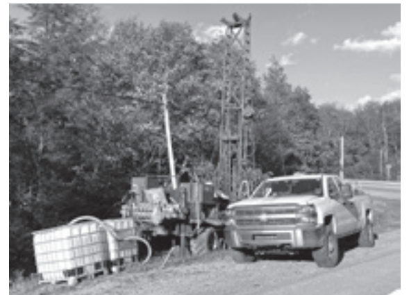
Core Drilling Begins off Rt. 219 at High School
